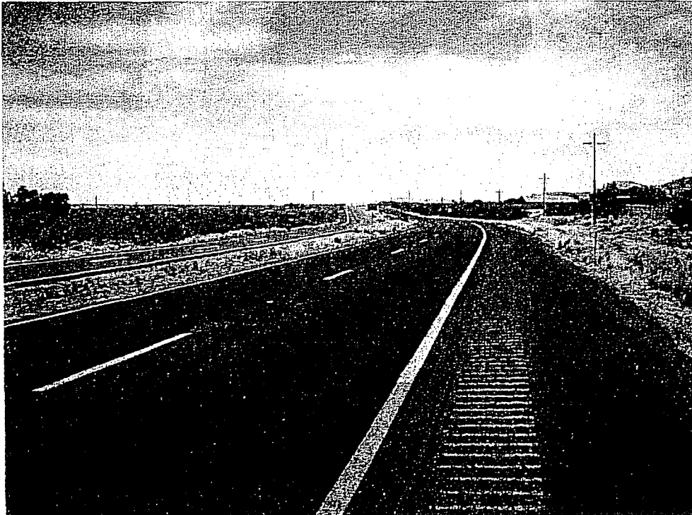
Photo 1: Street scene looking north on Oracle Road
