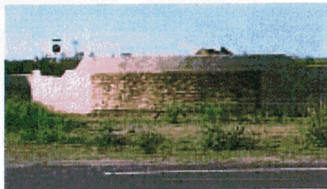
7.5 Example of preferred finish on perimeter fence.
