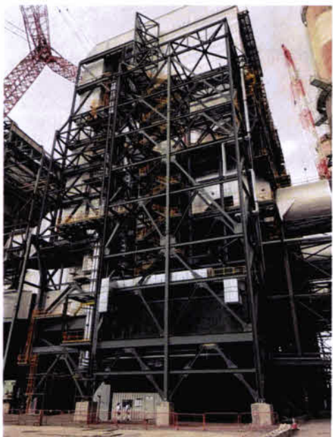
Unit 5 SCR Support Structure
