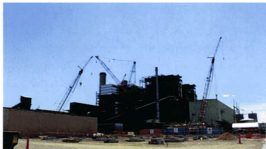
16 Unit 4 SCR Tie-in Outage Construction 17
