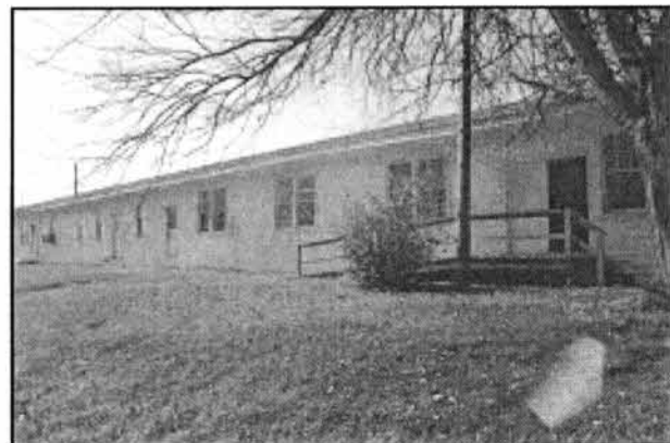
Figure 14. A side view of the exterior of the Center for Applied Technology, Cartersville.
