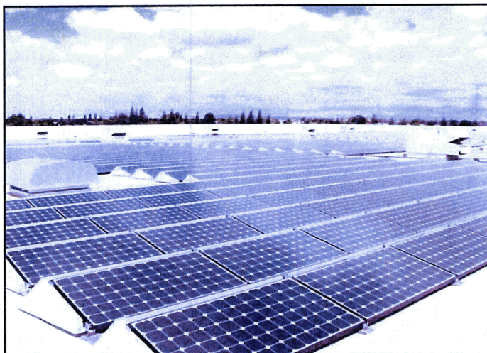
Figure 2-10: Solar Power System involved in April 2009 CA Incident 44
