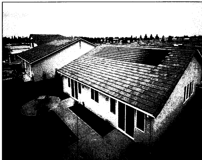
Figure 5-2: Residential Occupancy with a PV System Integral to the Roof Assembly (Photo courtesy of NREL Photographic Information Exchange)
