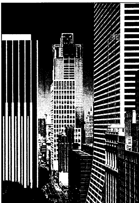
Figure 3-7: BIPV System Using a Vertical Module Configuration in New York City (Photo courtesy of NREL Photographic Information Exchange)
