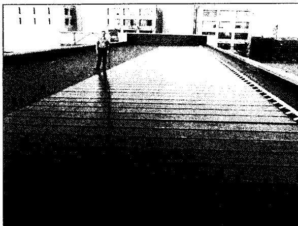
Figure 3-6: Example of Thin Film PV System on a Commercial Building in Detroit, MI
